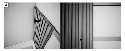
Mounting to the carcass is carried out by driving glass nails through the profile gaps.
