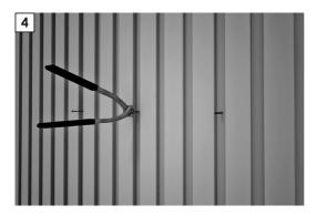
The visible heads of the nailed nails are cut with the help of pliers.
