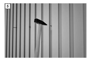
Then it is entered into the profile with the help of a hammer. Or instead of this whole process, a headless nail gun can be used.
